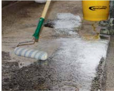
The underground surface must be primed with **PowerGrip** before further coating to create an optimum bonding bridge. To do this, mix the 2 components of **PowerGrip** homogeneously, decant in fresh bucket, mix again and then apply with a roller. **Let the primer dry.**
