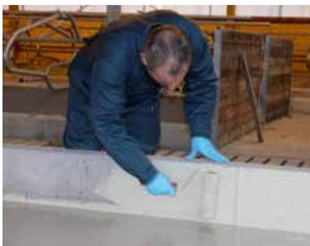
After priming, apply **Top-F** to the concrete back walls of feed tables and silo walls with a roller.
