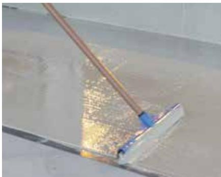
Apply **Top-F** to the feeding table and spread with a rubber squeegee, let the milling groove fill with **Top-F**. Finally unroll with a short pile roll.
