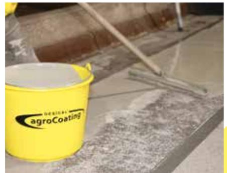
Mix the 2 components of **Basic** homogeneously and then **transfer** into another bucket and **mix again**.
