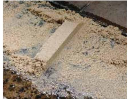
Very severely damaged floors must also be pre-filled with **easyFill** before coating with **Basic**. This creates a flat surface and saves material and grinding work. Mix the mineral mass with resin and hardener in a bucket. Apply the compound with a spatula and a smoothing trowel. For good compaction, tap firmly.
