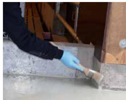
Apply **Top-F** to edge areas with a brush, if necessary paint over several times.
