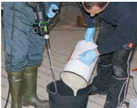
Mix the 2 components of **Top-F** homogeneously and then **transfer** into another bucket and **mix again**.
